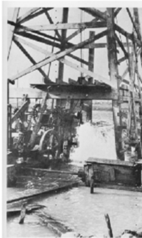
Pigs like this were used around the turn of the century to dig more than 1,000 wells into the 500-foot sand below Memphis.
